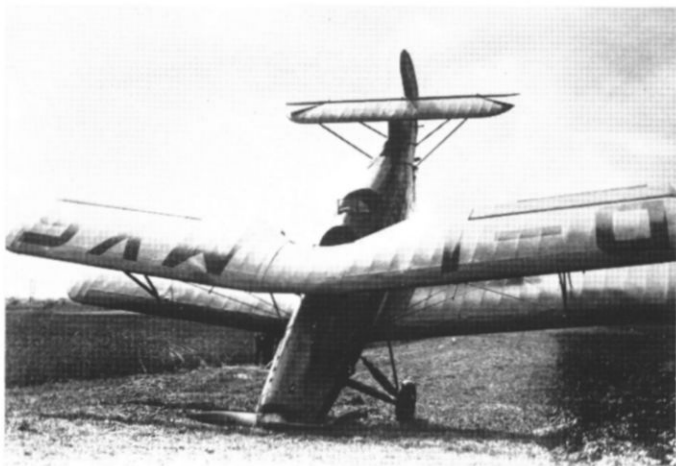
Left. This upended Arado Ar 66, photographed in the summer of 1936 at the Fliegerübungsstelle Freiburg , was a good example of the way civil registration was painted on training aircraft during this period. The color scheme was overall greenish-grey 63 and the registration letters were black. Right. Another Arado Ar 65 from the Schlessheim training school, showing clearly the white band around its fuselage, five-letter registration and in this case an entirely black propeller with a metal-sheathed leading edge.
