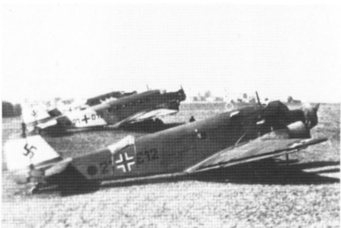
Left. On this Henschel Hs 123, CH+?W, white 5, the old background to the swastika had been overpainted and it is therefore safe to say that the photograph was probably taken during 1939. This aircraft carried the usual four-color camouflage and its underwing crosses in a most unusual inboard position. Note the small white letter L within a white circle just behind the cowling gills. Right. The use of a solid black disc beside the fuselage markings of these Junkers Ju 52s is something of a mystery, this photograph showing 21+D12, 21+E12 and 21+H12, all with the symbol. The difference between the four-color aircraft in the background and the more recent one in 70 and 71 dark green is obvious here.
