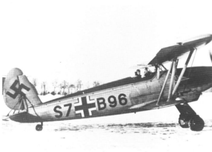
Left. Ready to go! This pupil awaits his instructor's signal to commence a solo flight. The Focke-Wulf 56 had the standard overall silver paintwork and a four-letter code. Of special interest is the narrow band, probably red, around the engine cowling, an unusual practice on this type of aircraft. The Focke-Wulf emblem under the wing showed a stylised eagle within a black-outlined disc which was probably light blue. Right. An Arado Ar 68 at Jüteborg in Spring, 1940, with an S7 code as described in the main text and grossly oversized swastika applied over traces of the former white disc and red band. The trainer had a dark blue top decking and thin piping. The paintwork had obviously been patched under the code.
