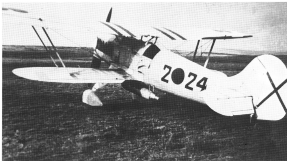
For a long time after the arrival of the first Heinkel He 51s in Spain, they wore their original pale grey color with full Nationalist codes and markings, but persistent recognition problems made changes a matter of some urgency. This example, 2024, carried two black discs on the upper surfaces of the top wing as well as four extra black stripes.
